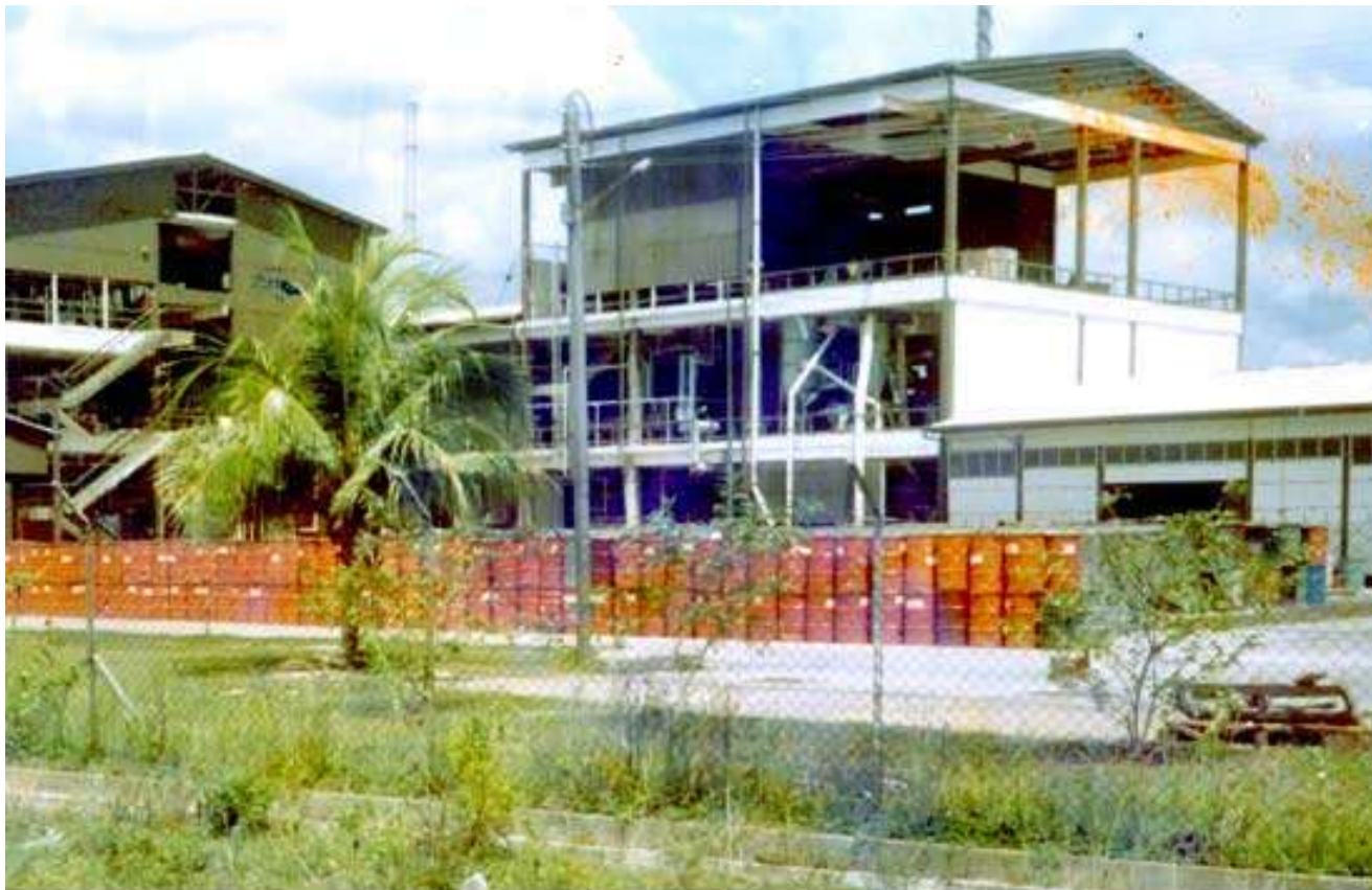
Asian Rare Earth in 1985. Note the drums of radioactive waste stacked in the open.
